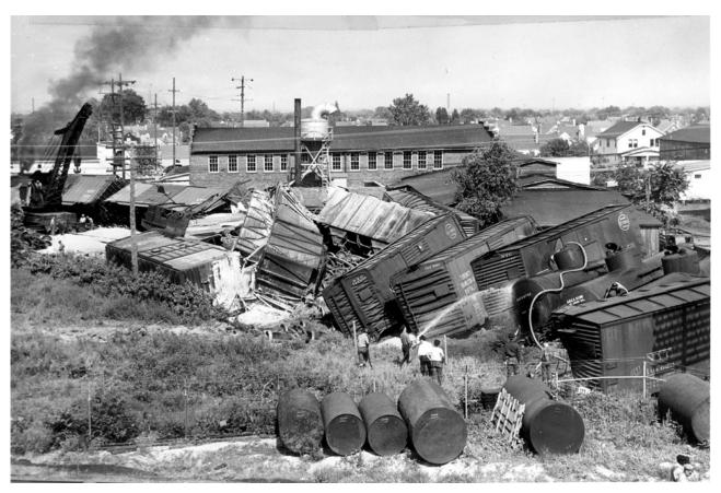
An engine and 22 freight cars were derailed on 5/30/1951 when an axle on one of the cars burned off. The wreck was located on the New York Central right of way immediately south of the West Broad Street crossing.
